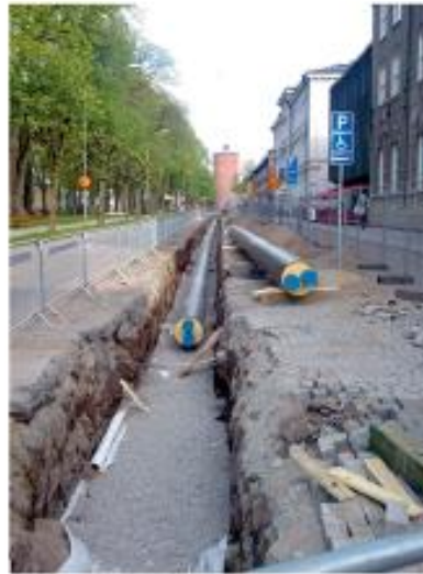
FIGURE 8.41 Left: Laying twin pipes joined within a trench. Photo: S. Werner. Right: Standardised trench. Source: Swedish District Heating Association.
